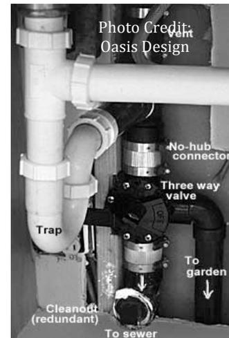
Each system must be custom designed to suit the building and the property. When all gray water sources are above ground level, a gravity fed system can be installed easily because storage tanks and pumps are not necessary.
